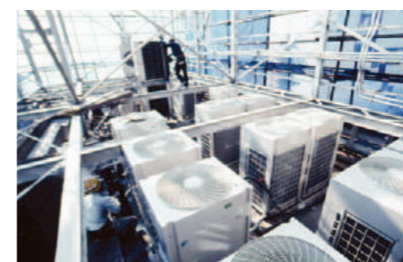
Replacement in progress
