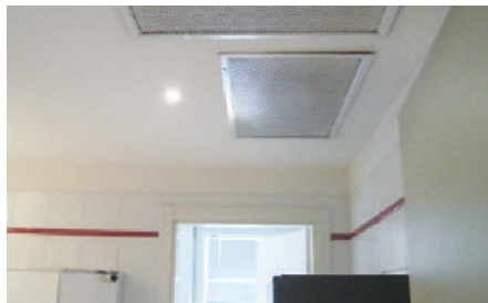
Installation was carried out during weekends to minimize disruption to business.
