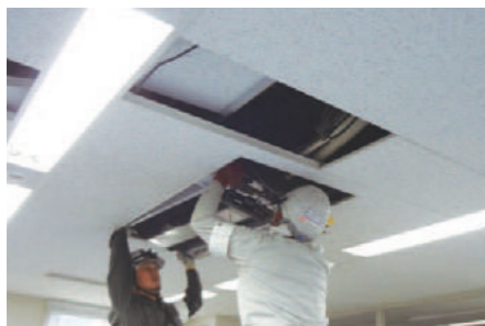
Removing old indoor unit
