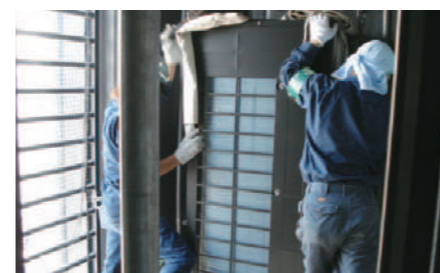
7 Outdoor unit installation
