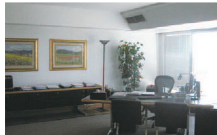
A VRV heat recovery system was installed on the top two floors which house a number of individual offices.
