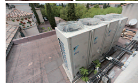
Replacement of the existing VRV system of a luxury 5 star hotel to anticipate R22 phase out while preserving interior decoration.
