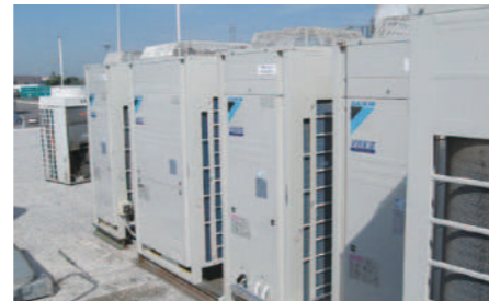
The VRV III-Q units run on R410A, ensuring compliance with the latest standards.
