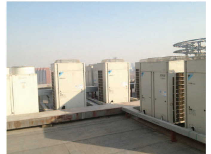
After VRV Q installation
