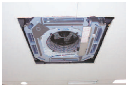
New indoor unit installed
