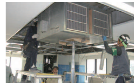
2 Removing existing indoor unit
