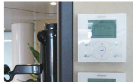
VRV allows independent control of climate in different areas of the building.
