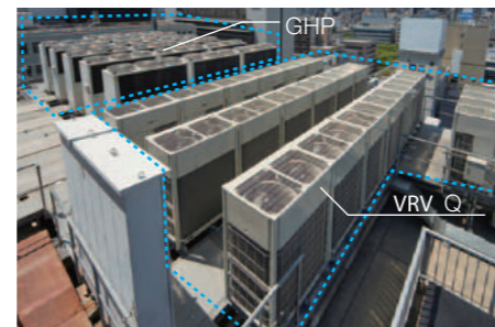
Replacement from GHP to VRV Q in progress
