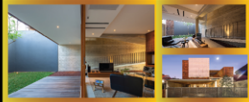
Project Gudang Peluru House ( Jakarta ) Designed by Wiyoga Nurdiansyah Architects AC Installed by Daikin Proshop AC System VRV HS and Multi NX
